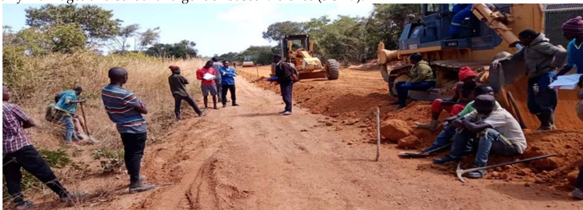
Workplace HIV sensitisations with road construction workers in Luwingu road: Photo –PEACE
